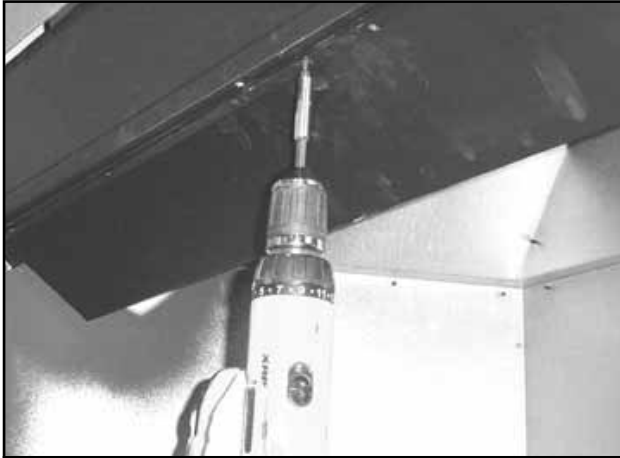
Figure 7.9 Remove Smoke Shield
