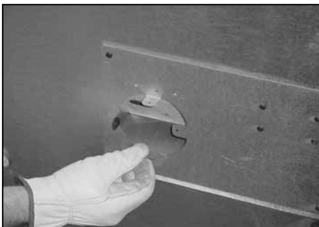
Figure 7.20 Bending Tabs on Outside Air Kit Collar
