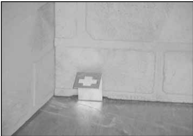
Figure 7.16 Grate Retaining Bracket in Place
