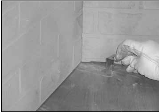
Figure 7.15 Slide Grate Retaining Bracket into Notch
