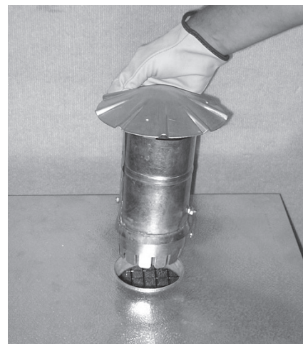
Installing the Chimney
