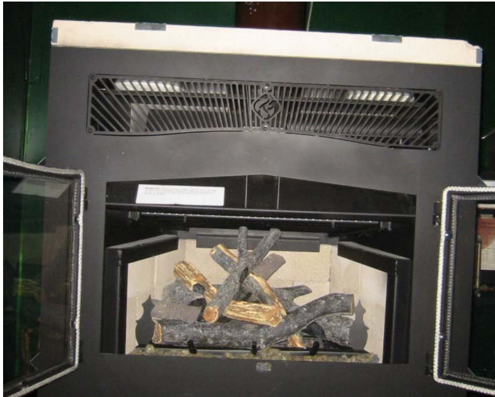
FIGURE 21: COMPLETED GAS LOG INSTALLATION
