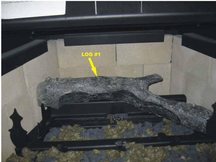
FIGURE 15: FIRST LOG INSTALLATION
