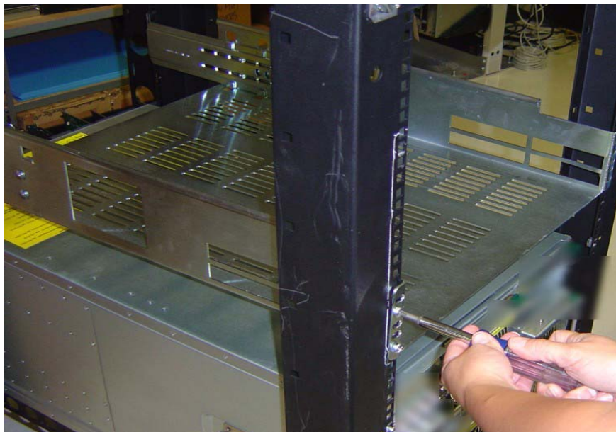
Figure 2-8: Screw the Shelf Ears to the Rack Posts
