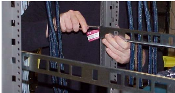
Figure 1-4: Secure Rack Brackets to Rack with Screws
