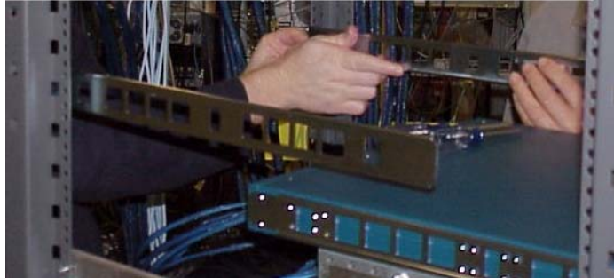
Figure 1-3: Holding Rack Bracket Against Inside of Rack
