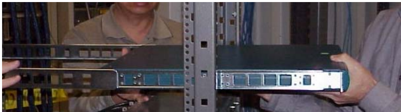
Figure 1-5: Sliding the Switch Into the Rack
