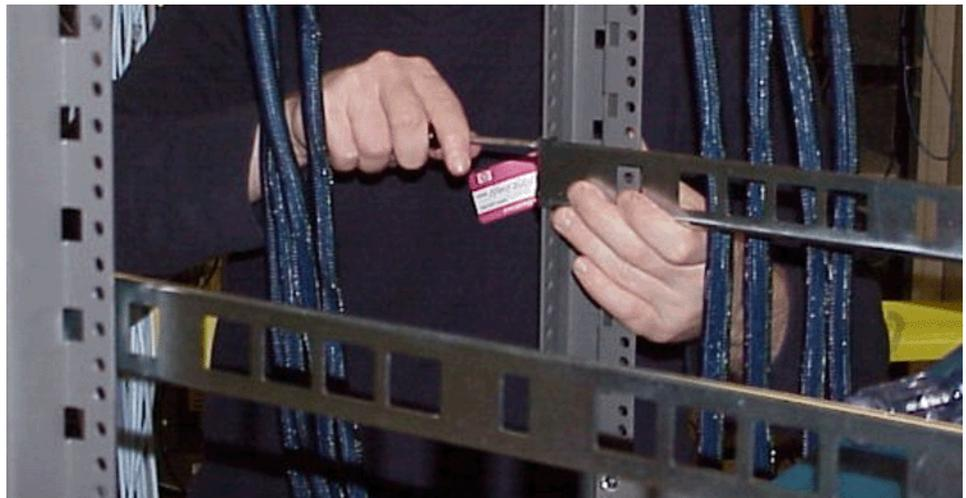
**Figure 1-4:** Secure Rack Brackets to Rack with Screws
