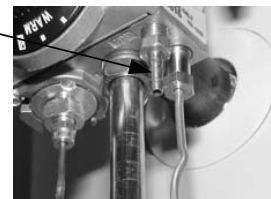
Pressure Tap Shown Installed
