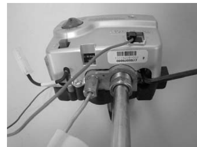
Gas Control shown in the "OFF" position
