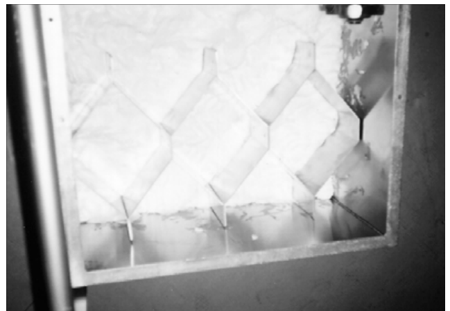
Figure 2-3. Installing the Cube Melter.
