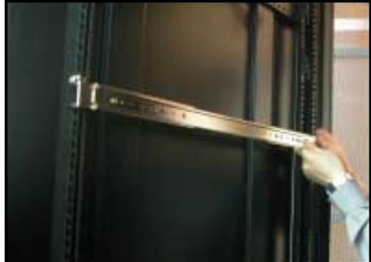
9. Secure the front end of the rail with two rack screws.
