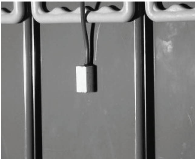
Figure 2.4-2 Battery Temperature Probe Installation
