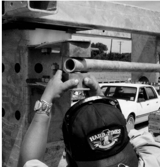
Figure 3-18: Azimuth Strut Assembly - Final Assembly
