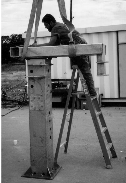
Figure 3-3: Raising Ground Mount Assembly
