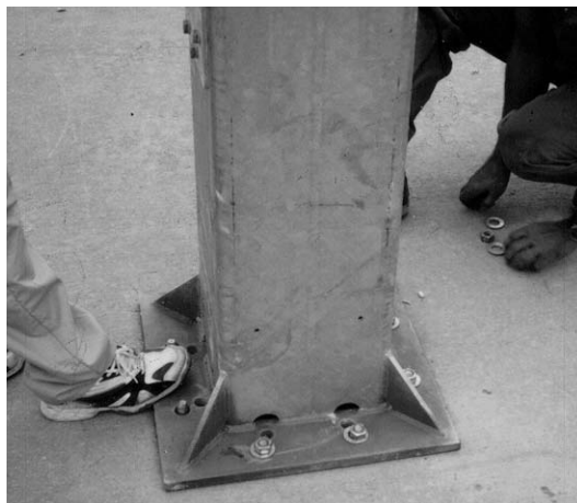
Figure 3-8a: Ground Mount Assembly Base Hardware
