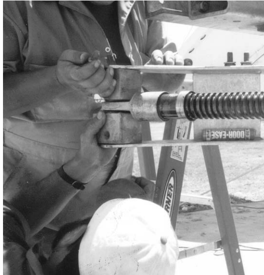
Figure 3-25b: Azimuth Jack Attachment
