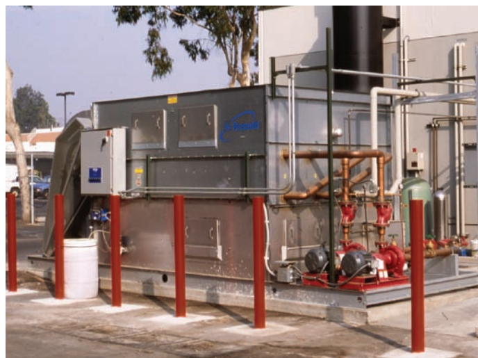
Recold JC Evaporative Condenser —Forced-draft, low profile design. G-600 galvanized steel factory assembled structure. Also available in 300 series stainless steel. Proven copper coil technology.
