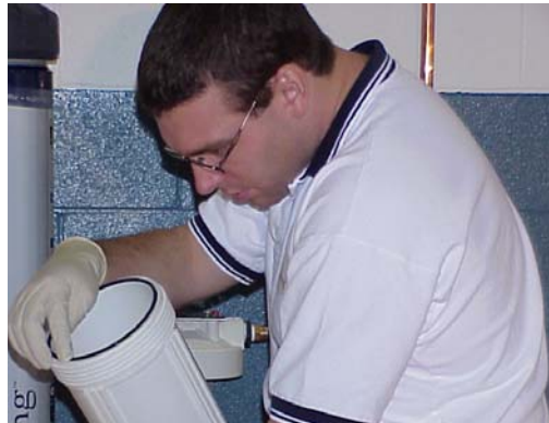
Photo 7. Inspecting o-ring.
