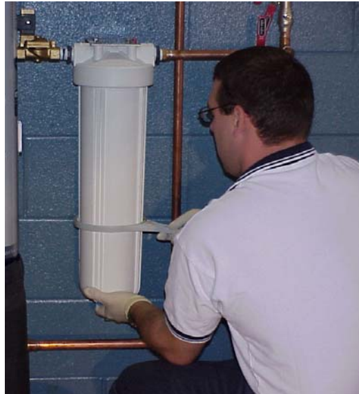
Photo 6. Disassembling the External Prefilter Housing
