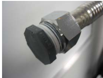
Photo 9. \frac{3}{4} ” Plug in Stainless Steel Flex Hose in Outlet Line
